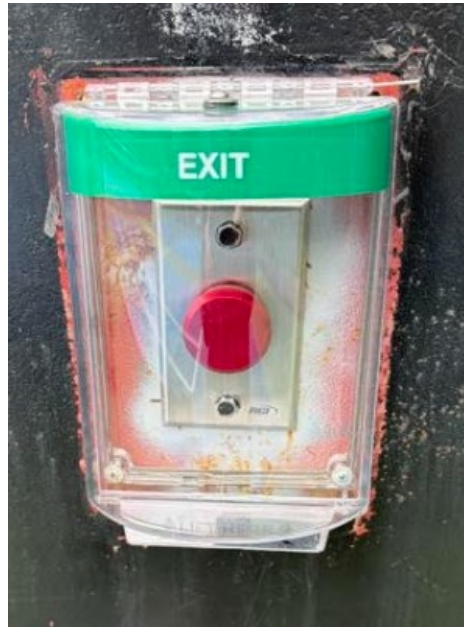
Exit Cover Replacement
