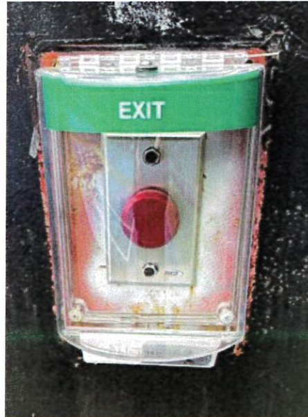
Exit Cover Replacement
