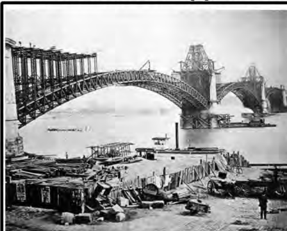
Eads Bridge during its construction
