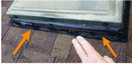
Sealant very dry and cracking, should be re-applied.
