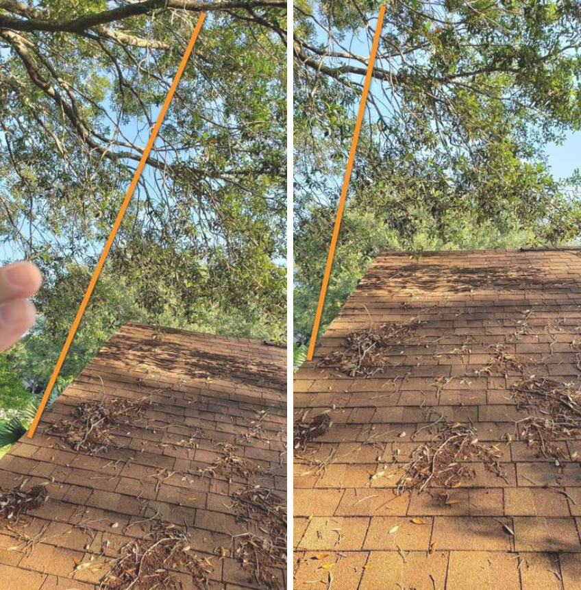
Trees should be kept from over hanging the roof. Trim trees from over roof.
