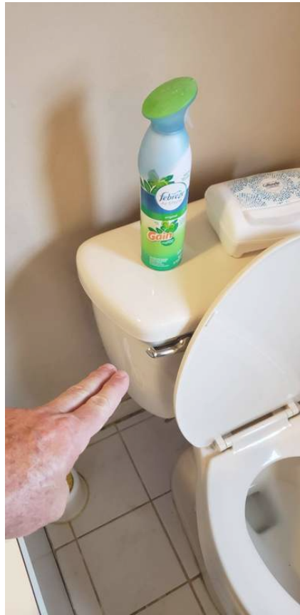
Tank needs tightening to bowl.
