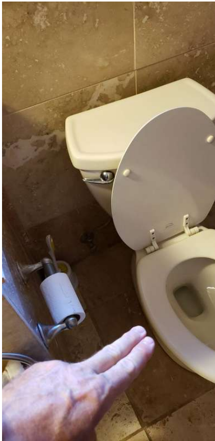
Toilet needs tightening to floor.
