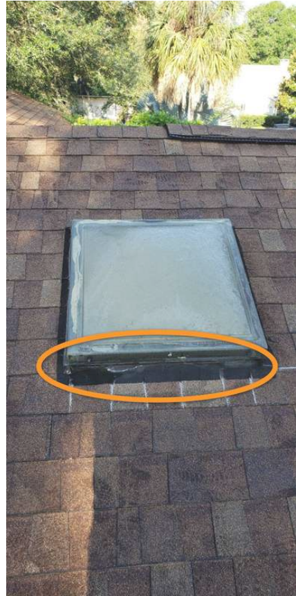
Re-apply sealant around skylights.
