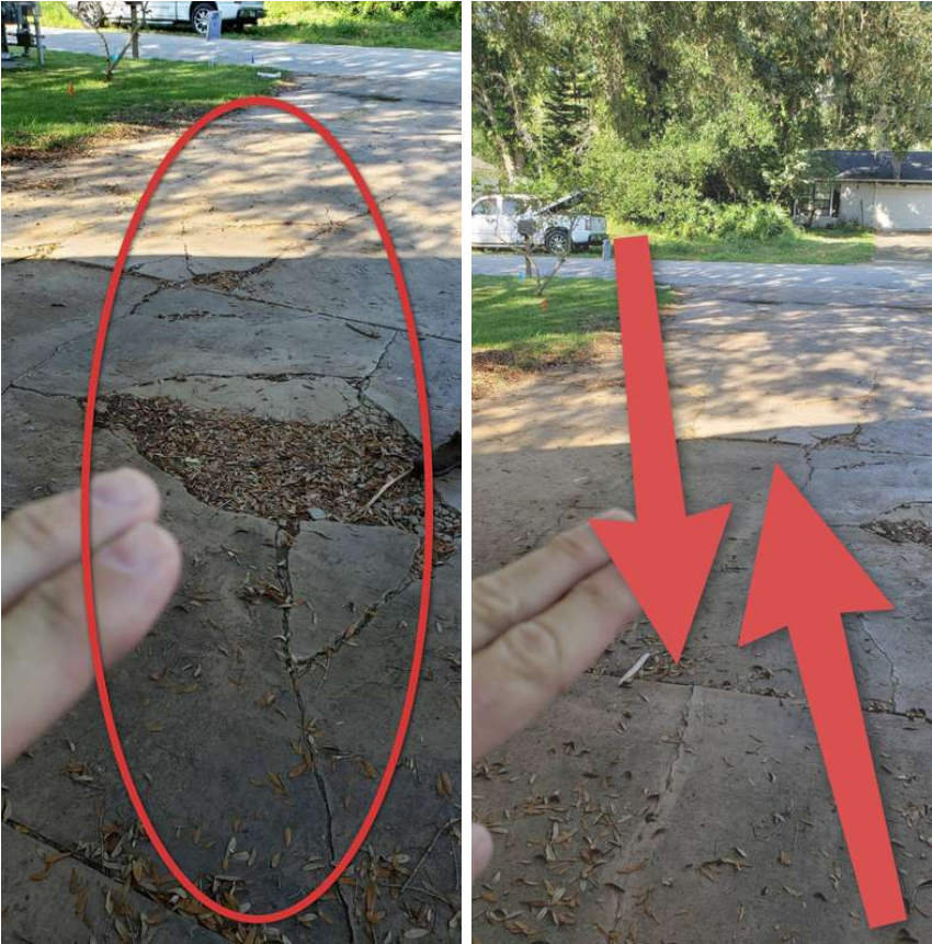
There are multiple major cracks in driveway. This is a trip hazard. These are safety hazards.
