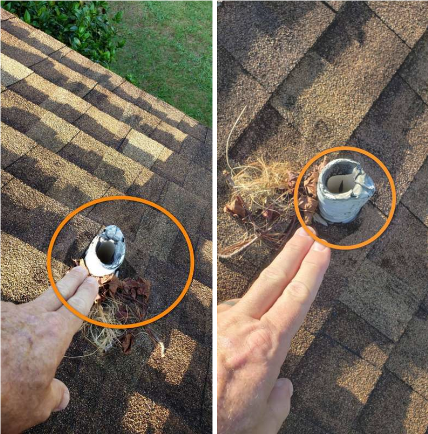
Lead sleeve needs to be repaired or replaced to prevent water intrusion. Lead sleeve needs to be repaired or replaced to prevent water intrusion.
