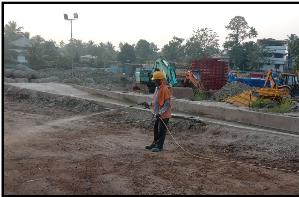
Photograph of the Water Sprinkling
