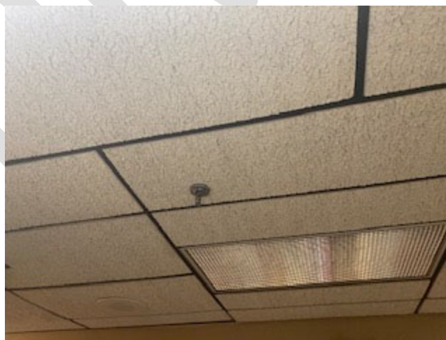
Sprinkler and Ceiling Tiles (Typical)
