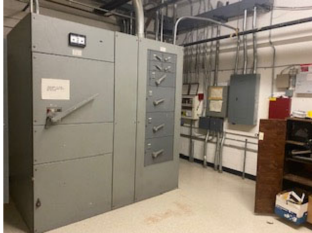
Main Electrical Room
