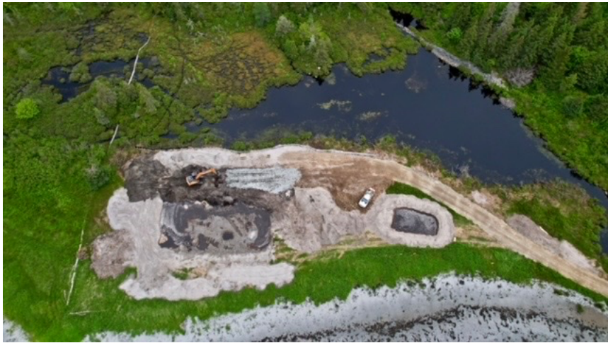
Photo of the excavation a week ago.
