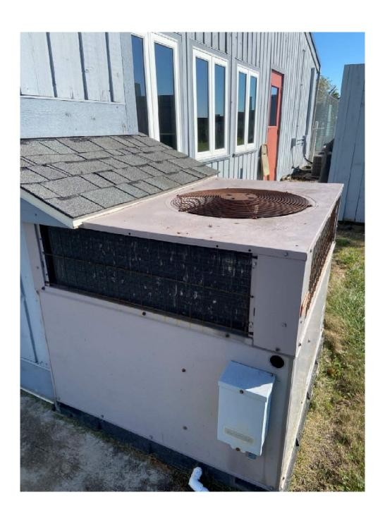
The outdoor air intake ducts for the main building HVAC systems have been capped and are no longer bringing in fresh air. New outdoor air intake ducts must be provided and routed through roof to meet current ventilation codes.
