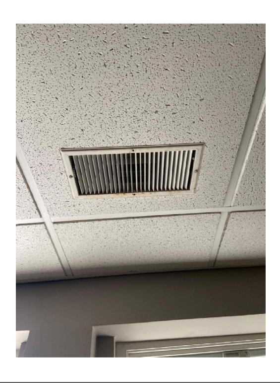
Gear and turnout storage rooms do not have dedicated exhaust. To meet current code, these rooms should have dedicated exhaust tied to a fan. Additionally, if the gear storage is moved out of the apparatus bay into a separate room, new exhaust will need to be provided for that room as well.
