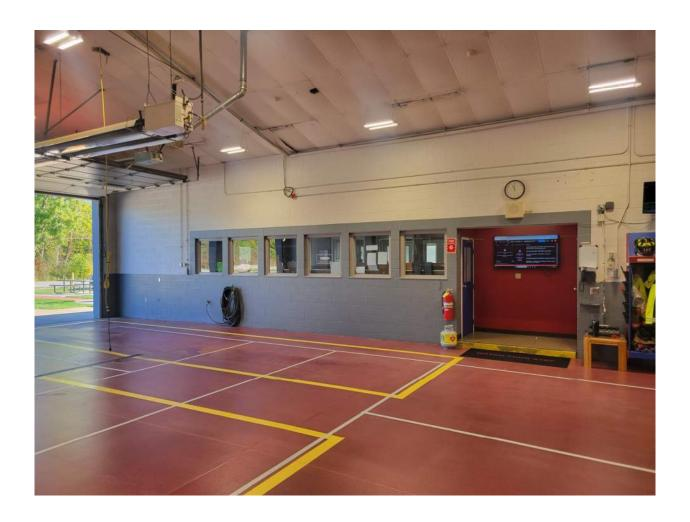
Acoustic ceiling tiles in this area of the App Bay are no longer flat and are visibly sagging in the grid. Many tiles are starting to grow mold as well.
