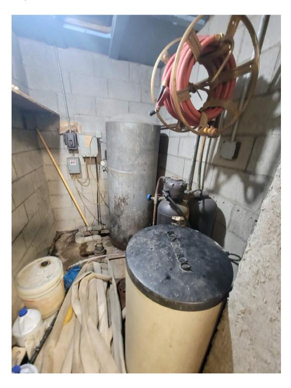
Domestic gas-fired water heater drain, now discharges into a bucket. Code requires a floor drain.
