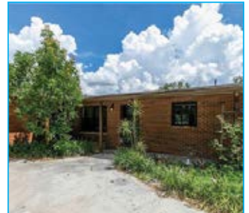
1262 SE Airport Rd
