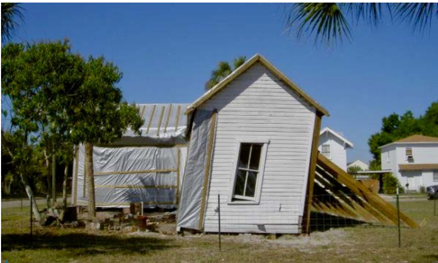
Hurricane Charley shoved the John Morgan Ingraham House Museum from its support piers, knocked down the chimney, and tore off much of the roof. Photograph courtesy of the DeSoto County Historical Society.
