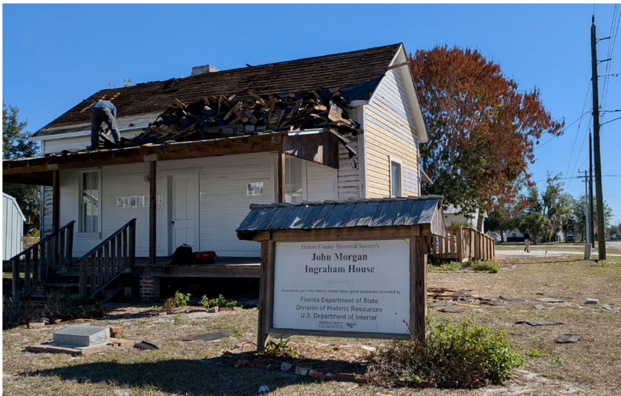
After Hurricane Charley and during the restoration funded by the State of Florida, Division of Historic Resources, wood shingles were installed on the roof, and when JSC Roofing stripped them off, the original purlins were revealed. Photograph courtesy of Carol Mahler
