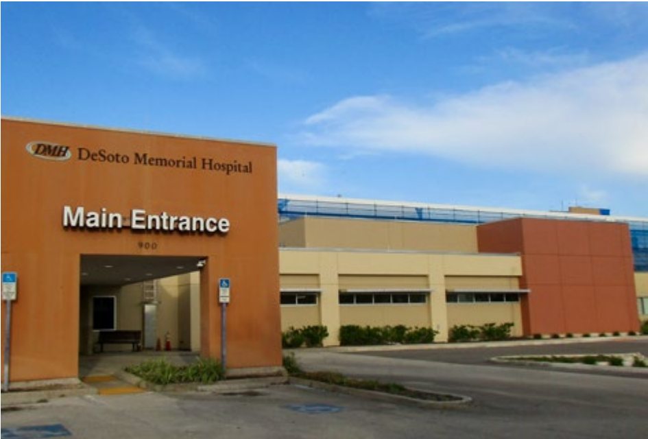
In July, DeSoto Memorial Hospital (DMH) was under construction for damage received during Hurricane Ian in 2022 with funding from the Federal Emergency Management Agency (FEMA) through the Florida Division of Emergency Management (FDEM). DMH Board Member and Council Member Bob Heine, Jr., announced that Tampa General has now leased DMH and will provide improved medical care in our community.
