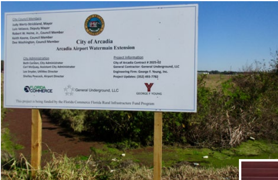
The Florida Dept. of Environmental Protection approved the City’s permit to extend the new airport water line into the Airport Estates subdivision, so residents may choose to connect to the City’s water service.
