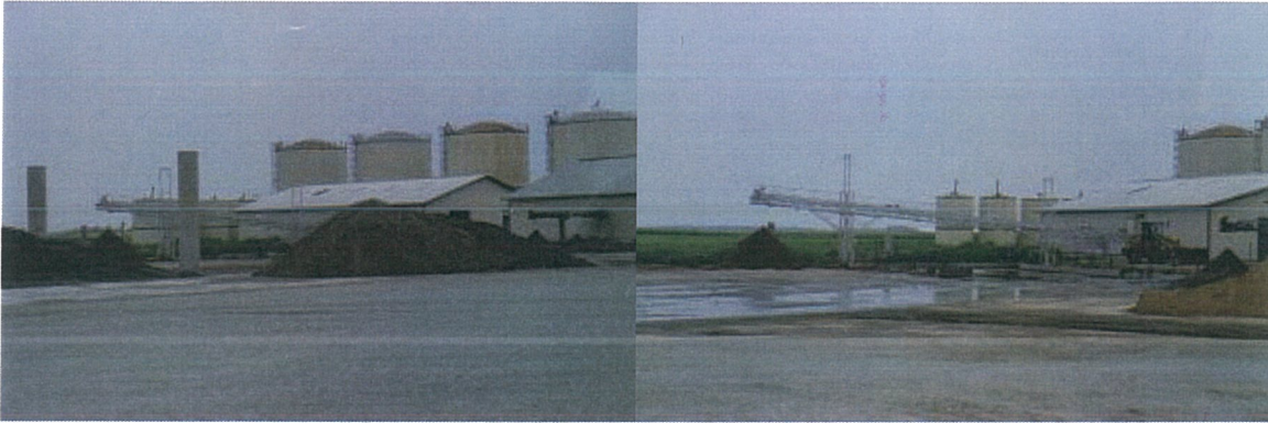
Plate 44-45: Anaerobic Digesters and manure separators
