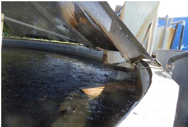
Fig. 3.9 Trickling tower is installed to remove CO<sub>2</sub> from the water
