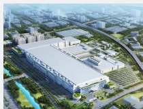
Display Foundry (显示面板厂)
