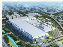
Display Foundry (显示面板厂)
