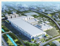
Display Foundry (显示面板厂)
