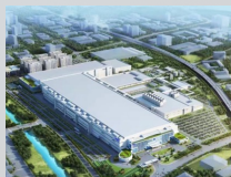
Display Foundry (显示面板厂)
