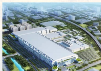
Display Foundry (显示面板厂)
