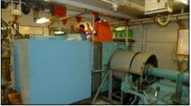
**Background:** Temperature alarms were triggered on one of the two 2000KVA shaft generators aboard the vessel. After discussions, the decision was made to put into harbor for diagnostics.
