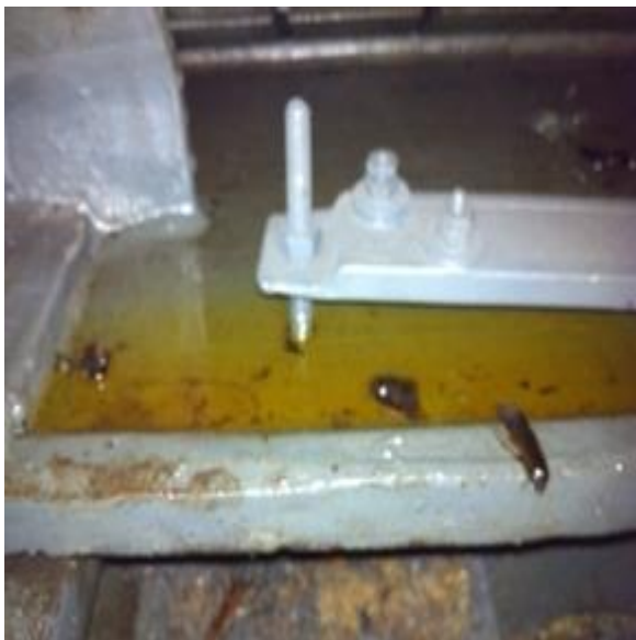
Photo of oil puddle in the motor base:
