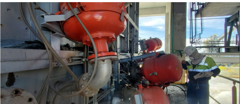
Figure 3. Air cannons often fail because of heat. Installations like this increase the heat and failure rate of any air cannon.
