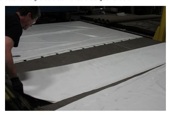
3. Roll the membrane no larger than 5 ft. 6 in. wide by 24 in. diameter. Ensure that the underside of the membrane is not contaminated with any foreign material as listed under **Requirements** on page 1.
