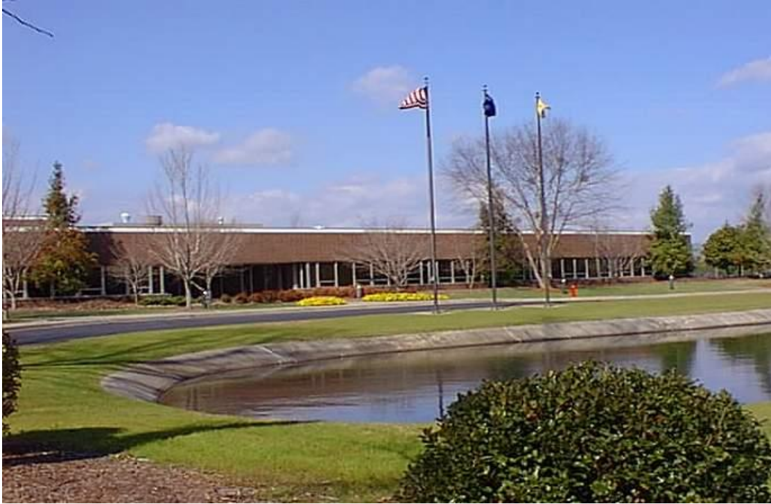
Bosch Anderson plant
