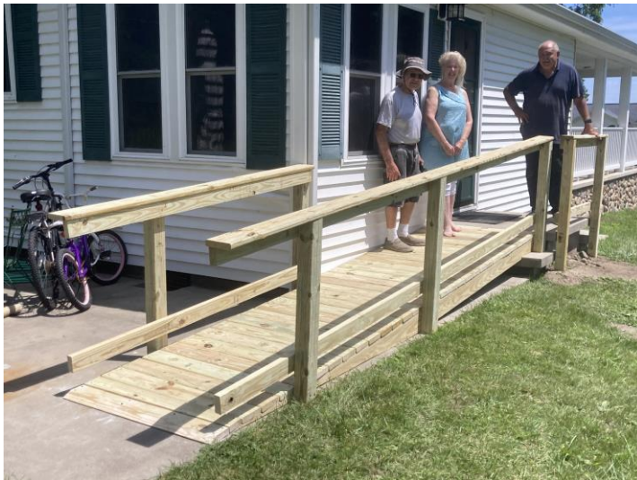
Harrisville Ramp – July 9th
