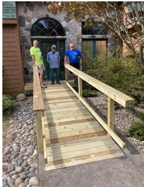
Oscoda ramp completed September 10 th .
