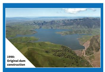
CAPACITY 100,000 acre feet **DAM HEIGHT** 192 feet **CREST LENGTH** 1,000 feet **CREST THICKNESS** 30 feet **BASE THICKNESS** 1,200 feet
