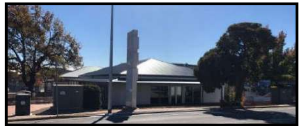
Above: The site of a new fitness studio in Littlehampton
