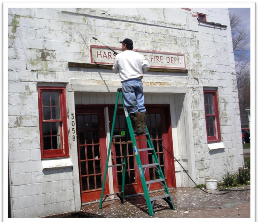
Powerwashing the exterior.
