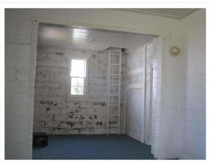
Interior shots after the walls were scrapped.
