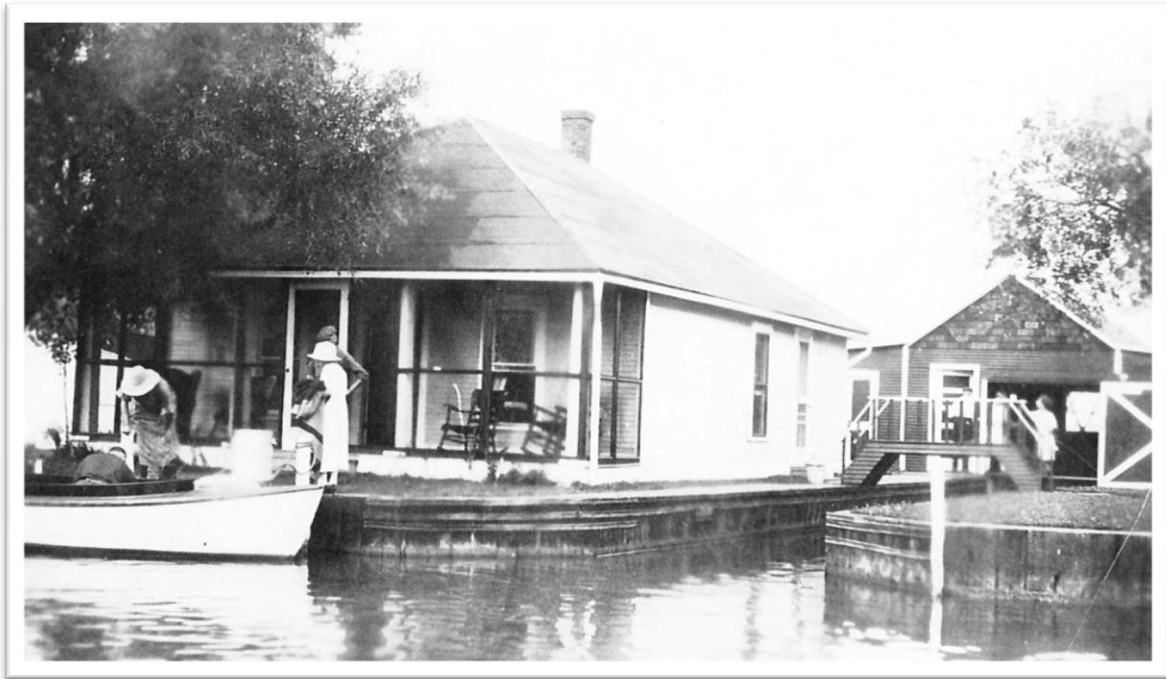
Picture 2, above: 7473 in the early 30's with a boathouse behind it, and a walk-bridge connecting the property to 7470. Wood sheet-piling, of course.
