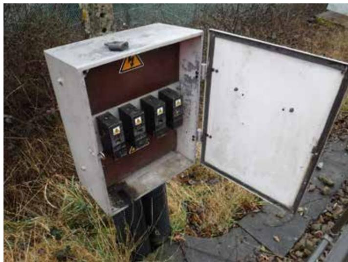
Existing joint/link boxes often contain a set of fuse carriers (the example above shows an extra set of fuses for a branch spur feeder). These are usually housed in a smaller steel enclosure mounted to an existing concrete or metal post. These existing enclosures provide an pivotal role in the isolation of feeder cables and segregated isolation.
