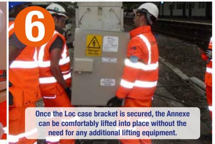
6 Once the Loc case bracket is secured, the Annexe can be comfortably lifted into place without the need for any additional lifting equipment.
