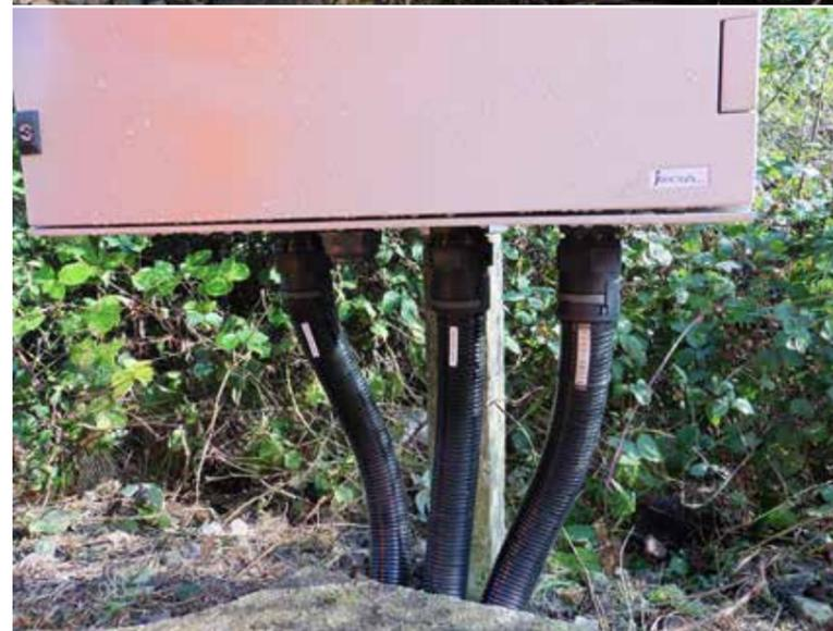
iLECSYS Rail have designed and manufactured a range of joint boxes that replicate the existing circuitry design. Joint boxes consist of a Micro FSP housed in a PADS approved GRP enclosure. These fully Class II joint boxes can be mounted to both existing and new posts using the innovative post bracket system.
