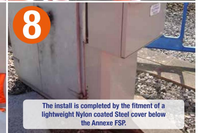
8 The install is completed by the fitment of a lightweight Nylon coated Steel cover below the Annexe FSP.
