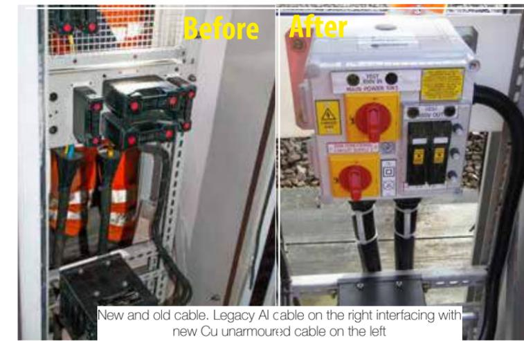
New and old cable. Legacy Al cable on the right interfacing with new Cu unarmoured cable on the left
