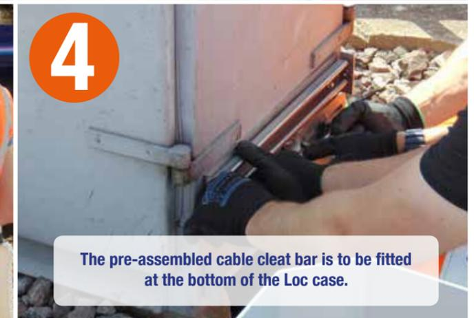
4 The pre-assembled cable cleat bar is to be fitted at the bottom of the Loc case.
