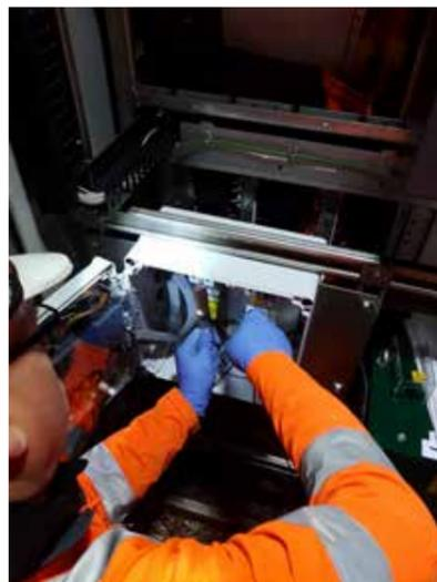
The larger Micro FSP complete with ESP was used on all installations. The larger tunnel terminals allowed for direct connection with the new Copper 2C 95mm<sup>2</sup> FGT cable.
