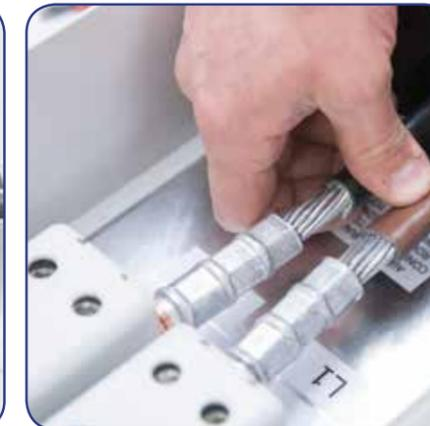
Cables are either directly mounted within the tunnel terminals, fitted with bi-metallic pins and located within the tunnel connections.
