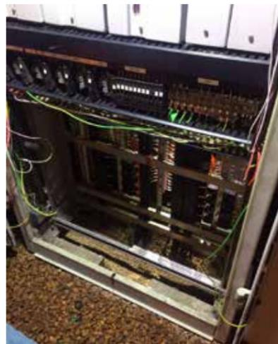
Starting from scratch. In some circumstances the quickest way to retrofit was to remove all of the existing equipment and re-build the location case. In this instance the install time was still kept to an impressive 2 hours 10 minutes.
