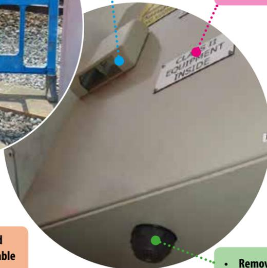
**GFRP Enclosure & LOC case mounting bracket.**
