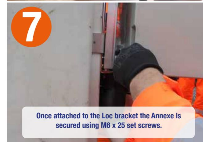
7 Once attached to the Loc bracket the Annexe is secured using M6 x 25 set screws.
