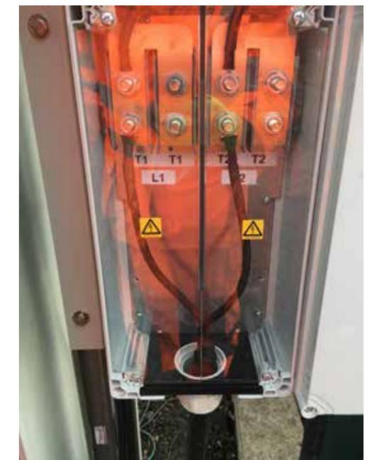
DITA Assemblies are supplied with large connection boxes to allow for the integration of 2C and 4C Cu and Al cable up to 150mm. A 3 core connection box is available for use with existing Class I Legacy cable. Connection boxes allow for the safe segregation of Class I and New Class II FGT cable
