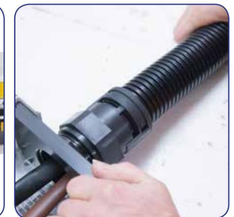
With larger sizes the conduit is secured within the gland using fixing clips
