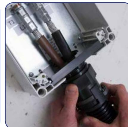
Incoming/outgoing feeder cables are tightened in place using approved conduit and glands. Glands can be attached to the pre-threaded plate without the need for locknuts.
