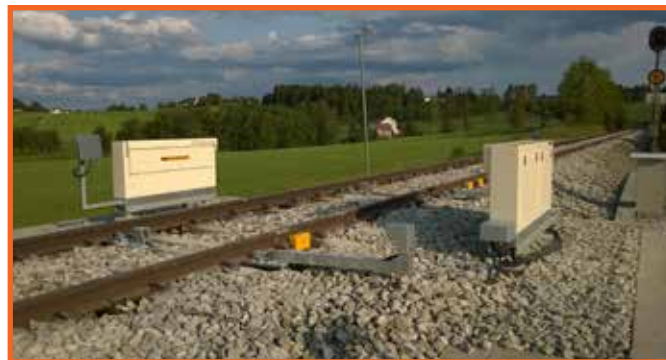
RailBAM and wheel condition monitor at Skatval, Norway.
