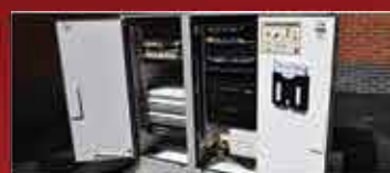
GSM-R/BTS-R/TEH Integrated Enclosures
