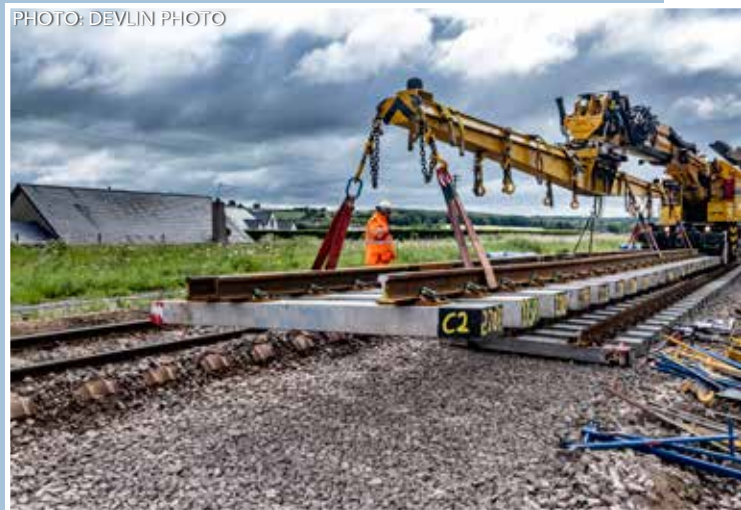
(Right) Kirow crane laying S&C at Inverurie on 7 July. (Left) Tamping new double crossover north of Inverurie.
