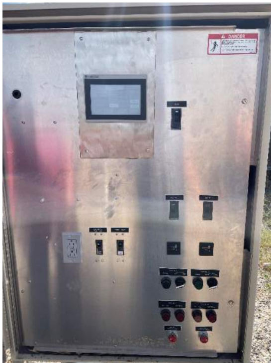
FIGURE 3-17: NORTH RESERVE LS CONTROL PANEL
