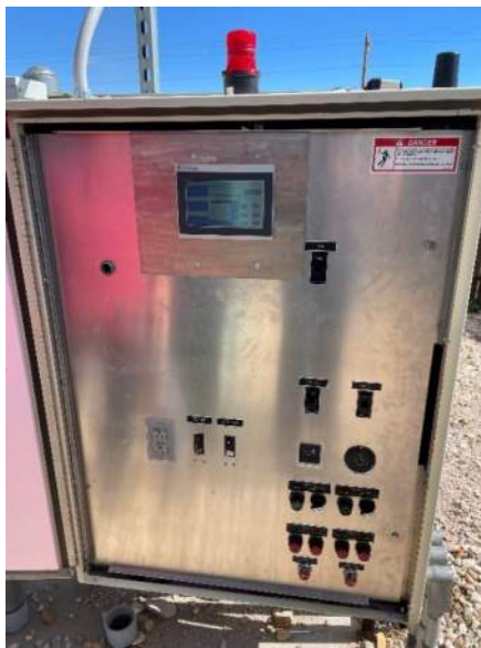
FIGURE 3-13: SOUTH RESERVE LS CONTROL PANEL
