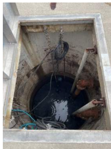
FIGURE 3-20: SUB #9 LS WET WELL
