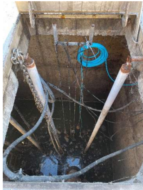
FIGURE 3-8: MAIN LS WET WELL
