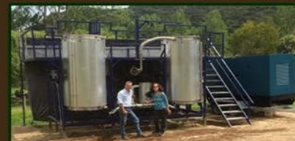
2021 - extraction plant, commissioned/ready
