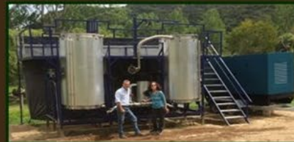
2021 - extraction plant, commissioned/ready
