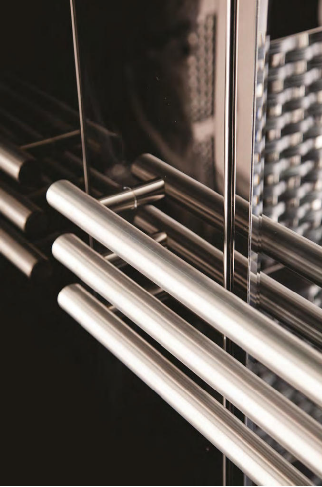
Figure 2: Rails such as these should not be attached to the car walls below a height of 800 mm.
