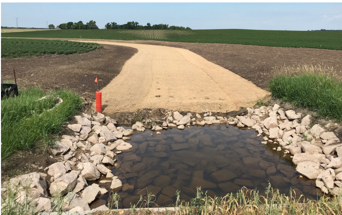
Pictured: An example of a field showing a newly constructed waterway.
