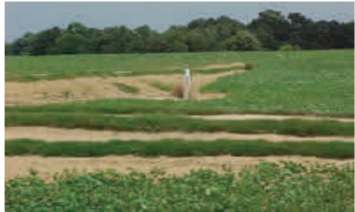
**Grassed Waterways** – This engineering practice involves constructing a vegetated channel that conveys runoff without eroding the underlying soil. The size and shape of a grassed waterway is based on the amount of runoff that the waterway must carry, the slope of proposed waterway, and the underlying soil type.
