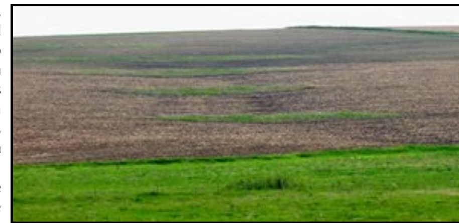
Looking upslope at a series of parallel water and sediment control basins built across a small watercourse on a cropped hillside. Photo courtesy MN NRCS.
