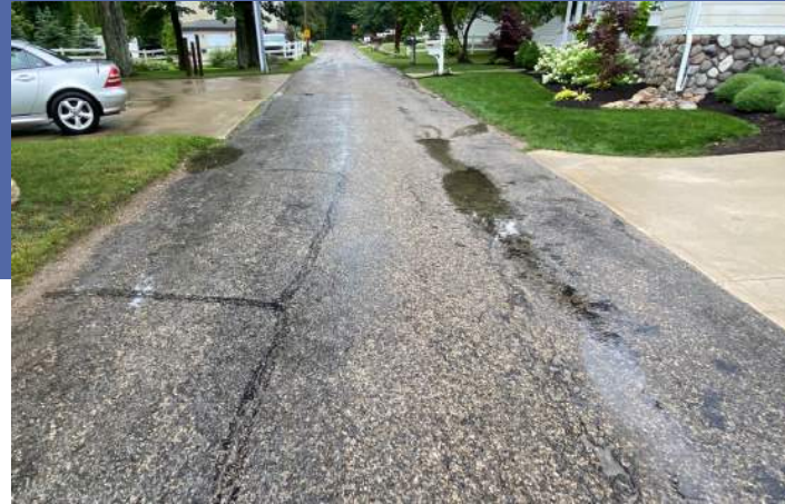
West Clear Lake Dr (Bridge to Lakeview)
