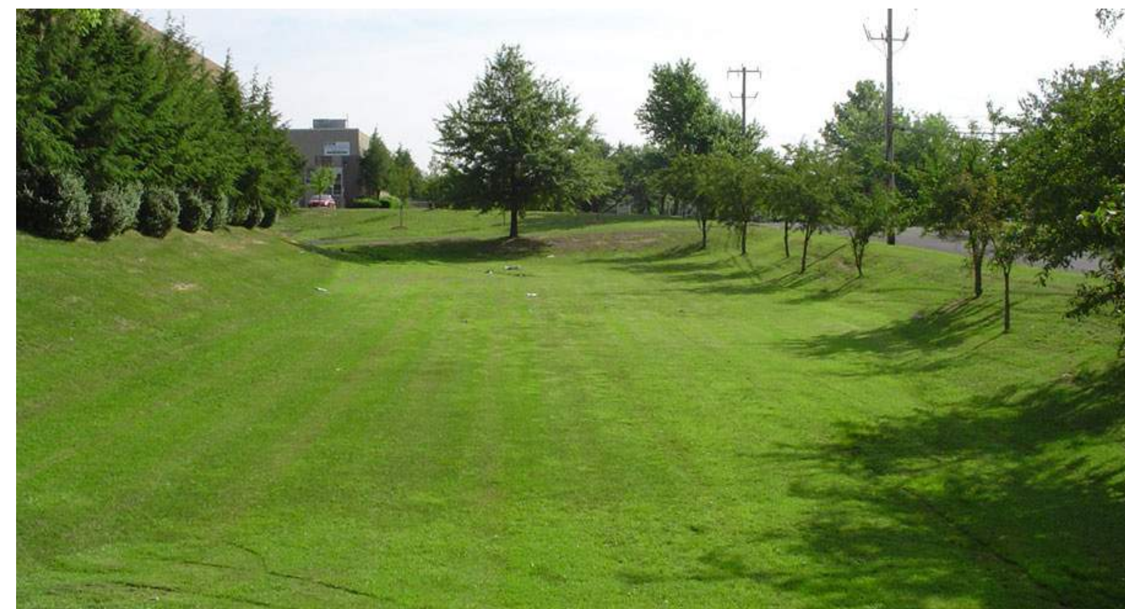
IMAGE OF A DRY DETENTION BASIN (TYPICAL)
