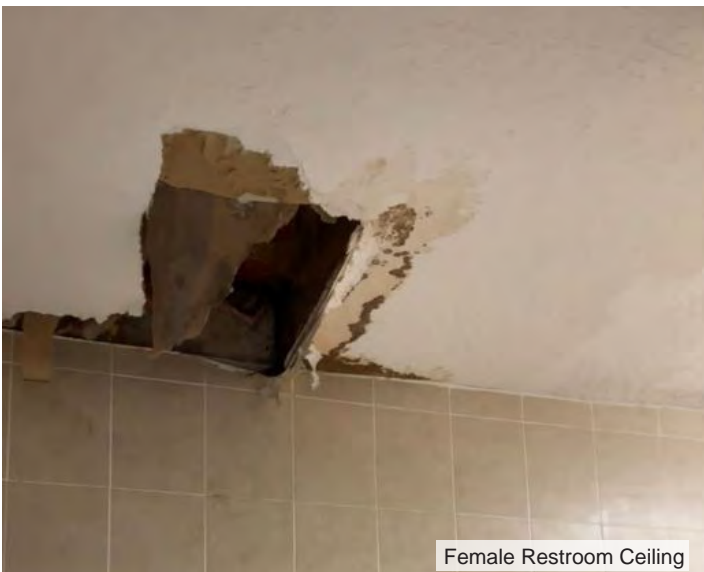
Water Intrusion Condition
