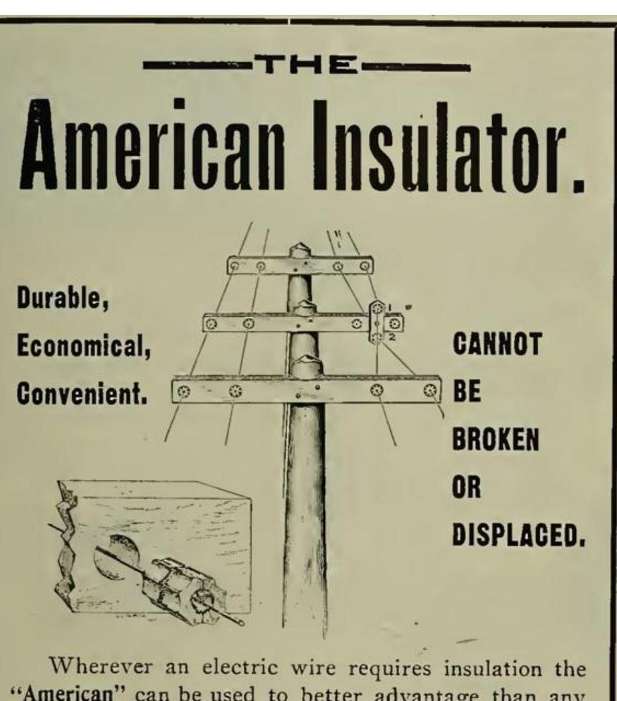
Wherever an electric wire requires insulation the "American" can be used to better advantage than any other. See practical demonstration of this device at the Convention.
