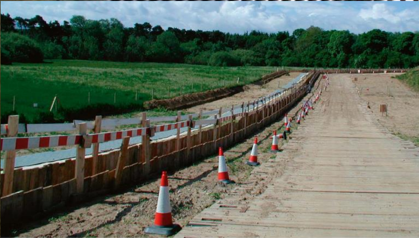
A cable swathe during construction with a single cable trench open
