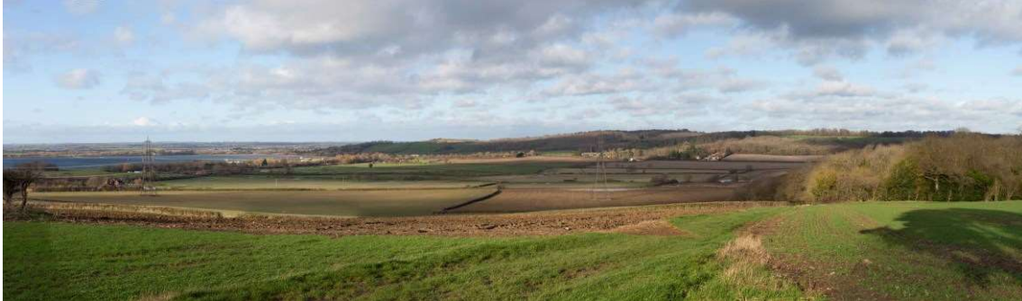
Botley West near Oxford would be the largest solar farm in Europe, covering 3,400 acres PHOTOVOLT DEVELOPMENT PARTNERS (PVDP)
