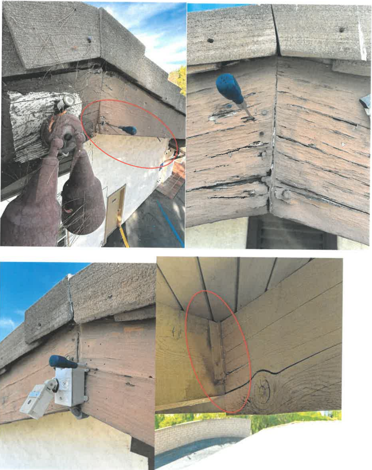
This picture shows the HU410 inverted hanger installation Note all pictures with dry rot. The extent of the owl is inside the wood is proportional to the damage.
