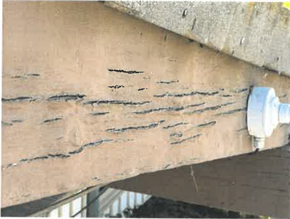
The paint no longer provides protection
