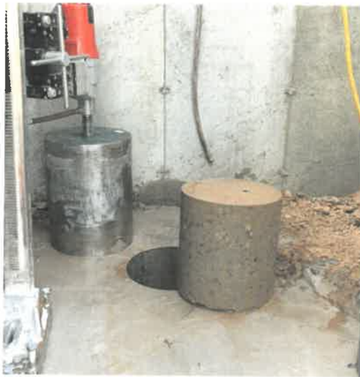
Typical core drilling
