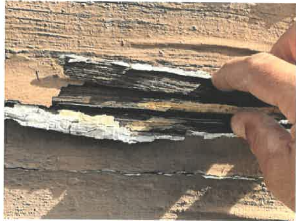
Previous repairs on cracks are deteriorating
