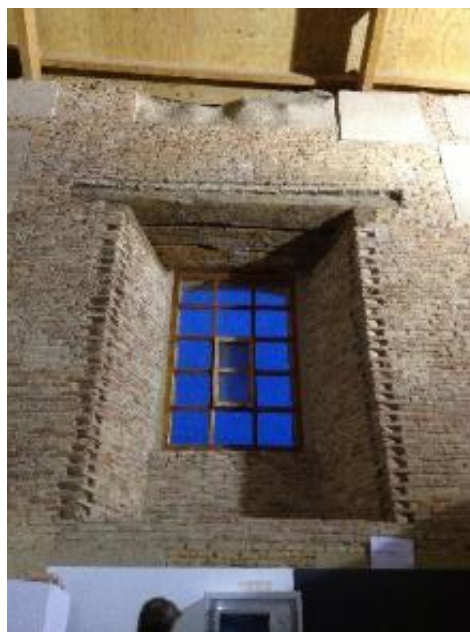
They put a roof on the old Monastery to make a bunkhouse
