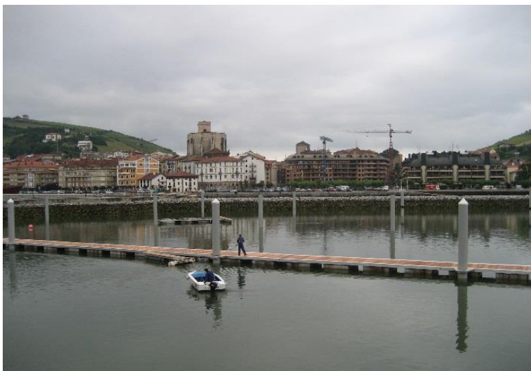
Just Building the Marina at Zumara
