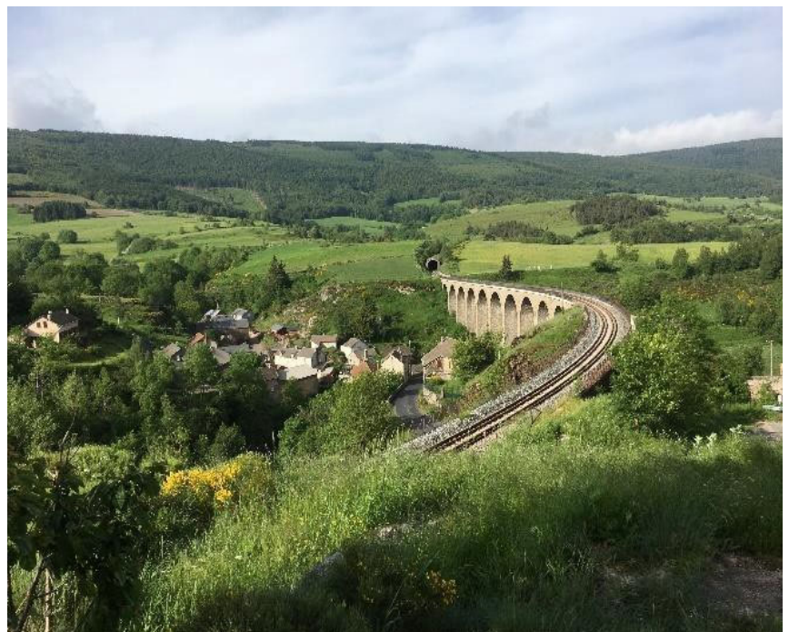
The beautiful Mirador Viaduct. Note snow tunnels
