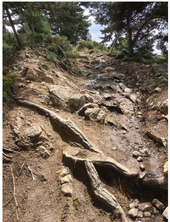
The storm damaged descent to Goudet gets worse
