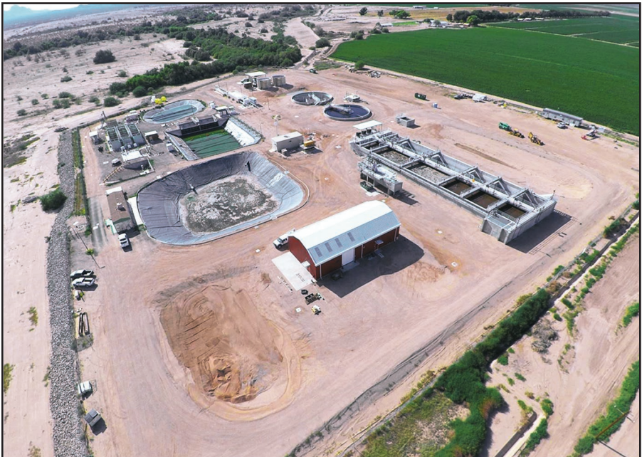
Marana Water Reclamation Facility.
