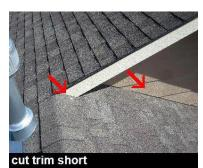
CONDITION: Missing flashing noted, unpainted area.(picture)
