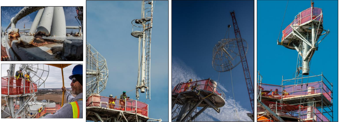
(Above) The Showboat's foremast was removed in three separate lifts. Once workers prepared the structures for removal, the crane swung in to first remove the upper section of the mast, followed by the SK-2 air search radar dish, and then the final section of the foremast severed at the platform just aft of the Forward Main Battery Director (Spot 1).
