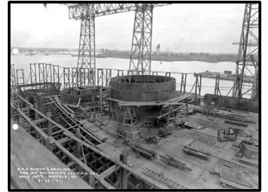
A view of BB52 under construction at Norfolk Naval Yard looking aft from amidships.
