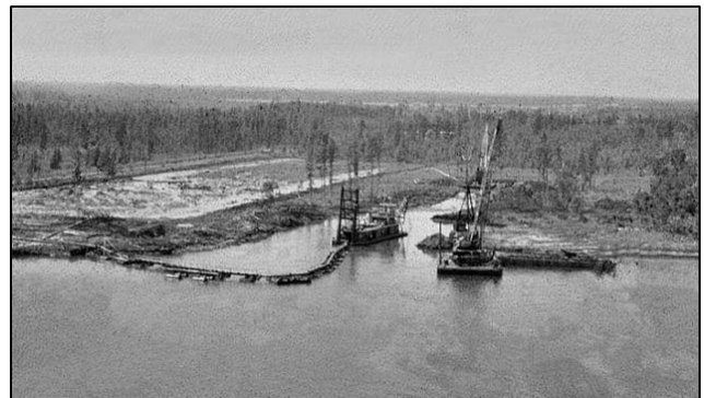
Dredging the site that will berth Battleship North Carolina .
